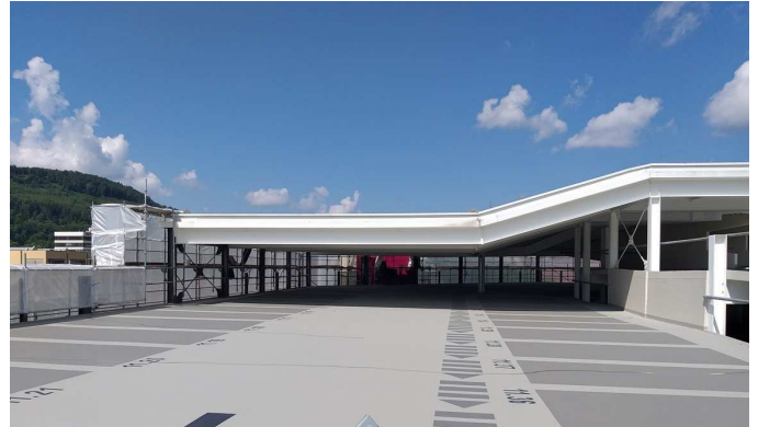
Roof level after restoration (Photo: Kerstin Götz)
