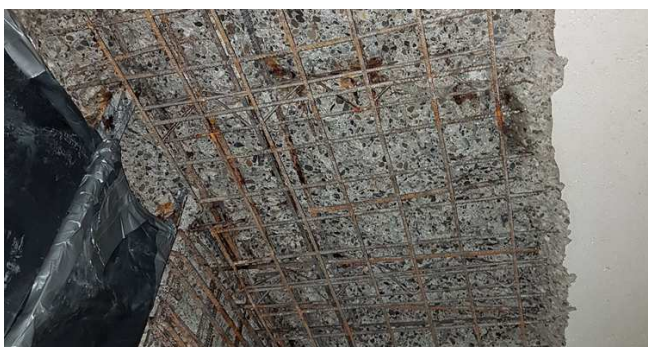
Rehabilitation of a damaged area (Photo: AMP)
