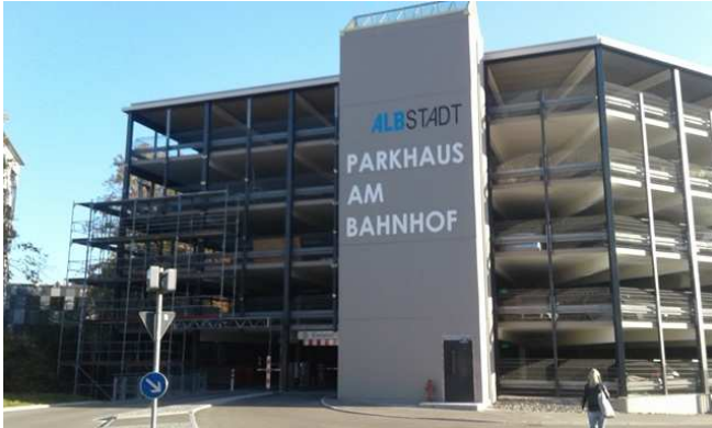
West Elevation, new ingress/egress (Photo: Kerstin Götz)
