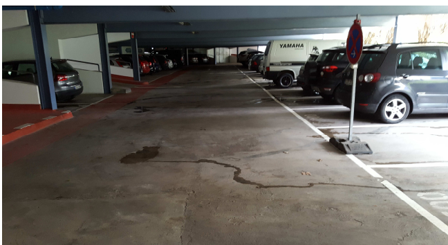
Parking level before restoration (Photo: AMP)
