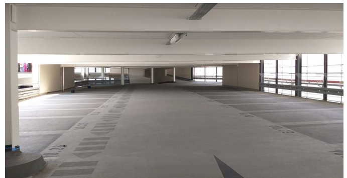
Parking level after restoration (Photo: Kerstin Götz)
