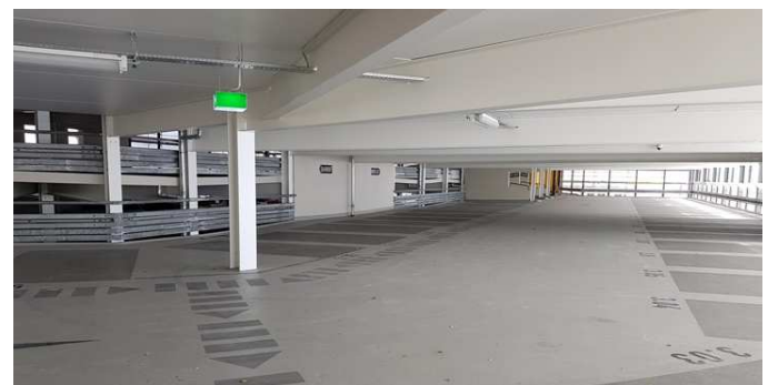
Parking level after restoration (Photo: AMP)
