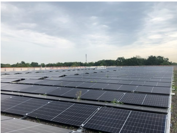
Roof view with photovoltaics (Photo: AMP)
