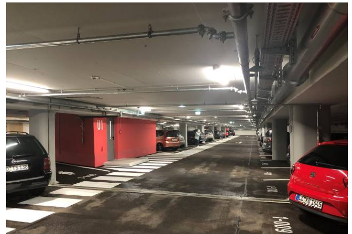
Car Park after renovation (Photo: AMP)
