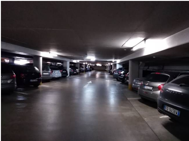
Car Park before renovation (Foto: AMP)
