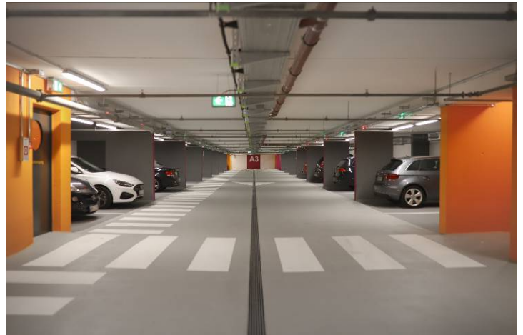
Car Park after renovation (Photo: Levin Liebmann)
