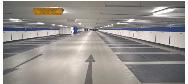
Parking Level 2 after renovation (Photo: AMP)
