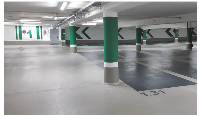
Underground level after restoration
