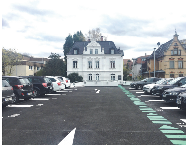
Open deck after renovation
