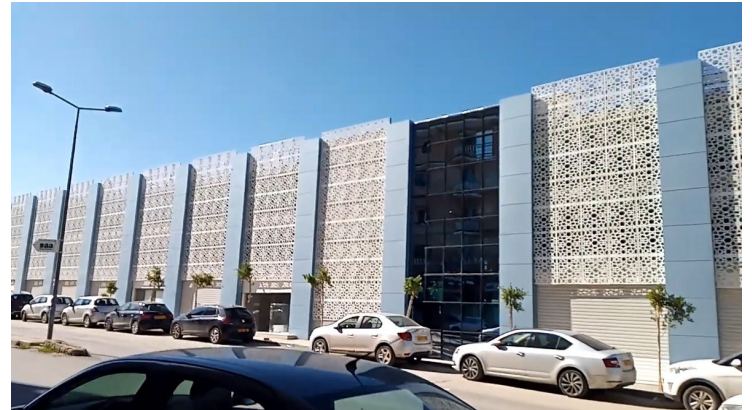
Facade view with shops
