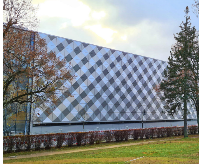
3D-Facade (Photo: AMP)
